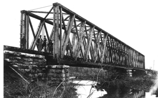
The Trace Creek trestle near Denver, Tennessee, on the Nashville and Northwestern R.R. in 1864. Library of Congress
